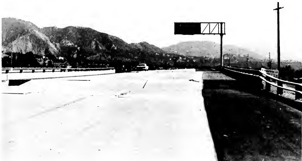
Photo 7. Settlement and offset of bridge approach fill on Route 210. Note ramp effect of approach slabs.
